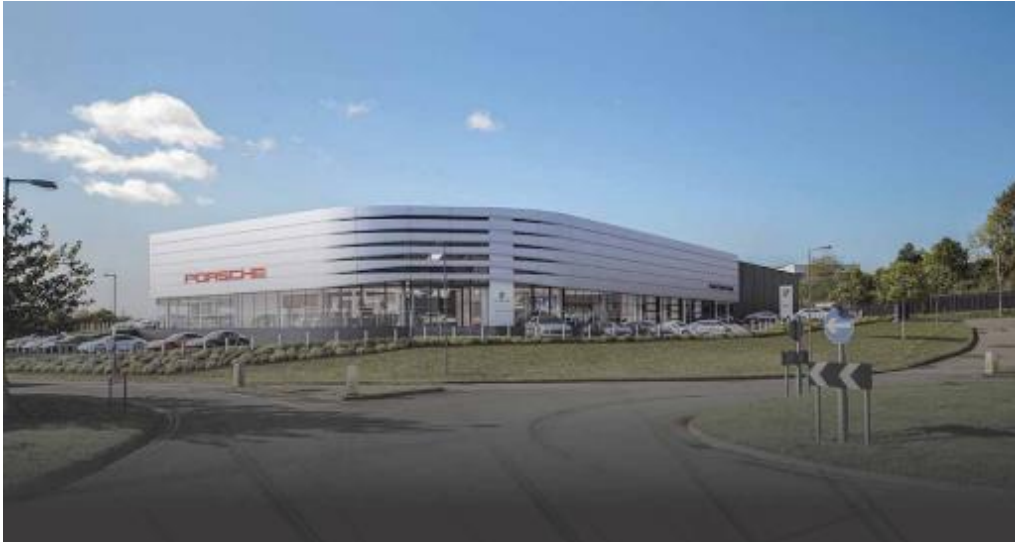
FIGURE 6: PORSCHE CENTRE LAND ON THE NORTH SIDE OF LAKESIDE DRIVE
