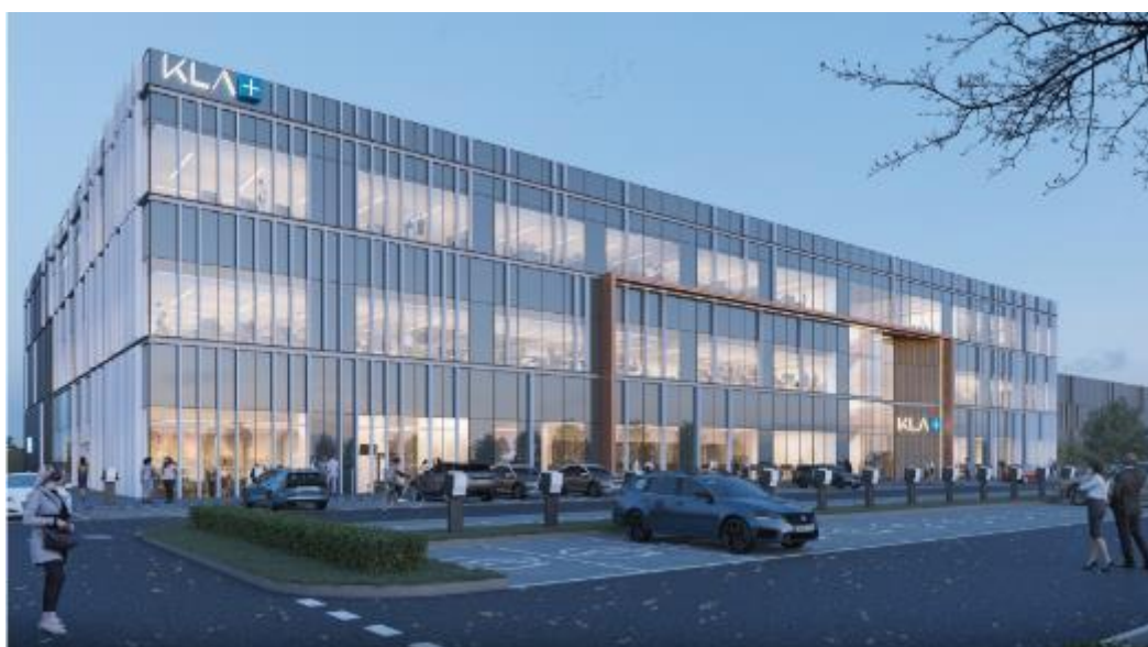
FIGURE 5: RESEARCH AND DEVELOPMENT FACILITY AT PLOT 1 AND 5, IMPERIAL WAY (EM1(i))
