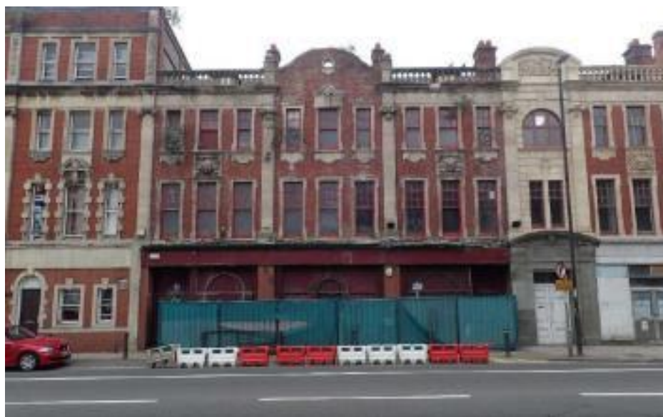
FIGURE 22: RESTORATION WORK TO GRADE II LISTED BUILDING
